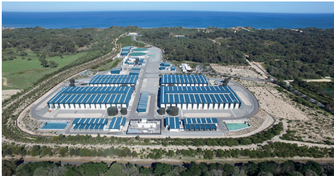
Perth Desalination Plant. Australia
