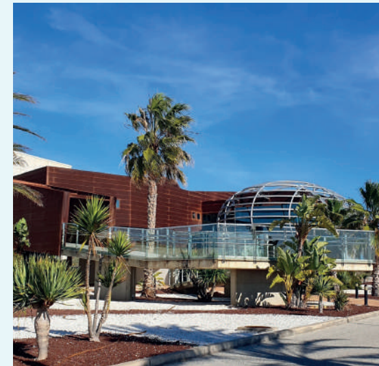
Life hyeward project. Alicante desalination plant. Spain
