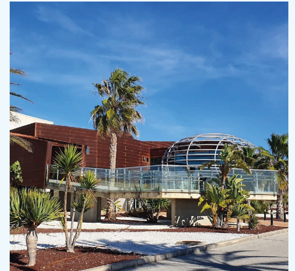
Life hyeward project. Alicante desalination plant.
