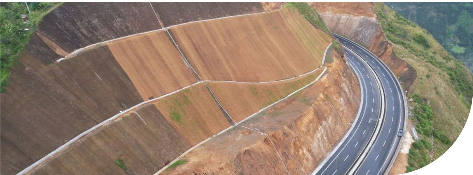
Intervention in the Rumichaca-Pasto Double Lane project (Colombia) with the installation of coconut fiber biomantle.
