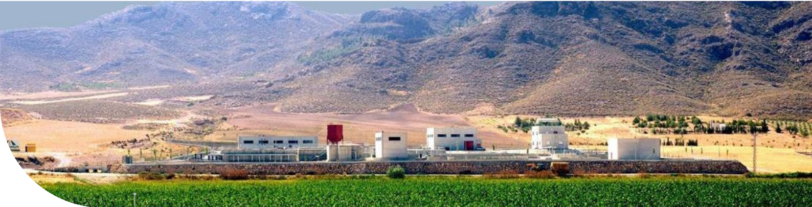
Jumilla wastewater treatment plant
